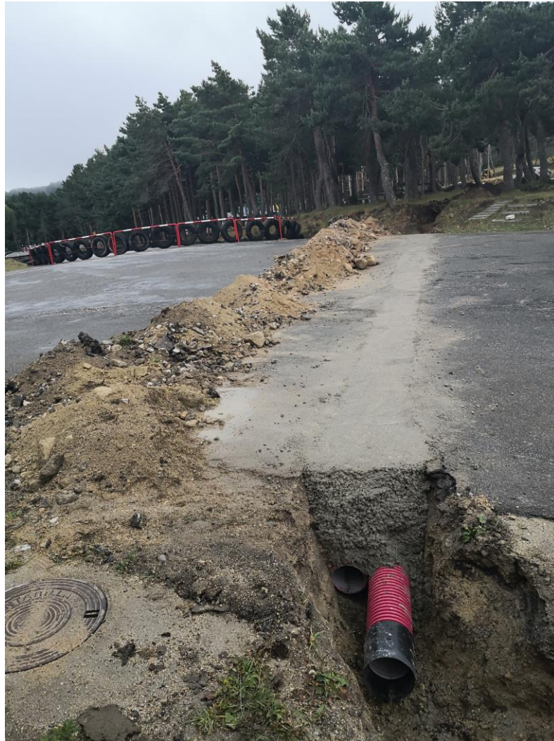
Figure 76- CT3 PV wiring in trench
